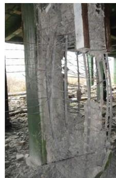
b) Concrete damage and rebar bending after the detonation of the charges
